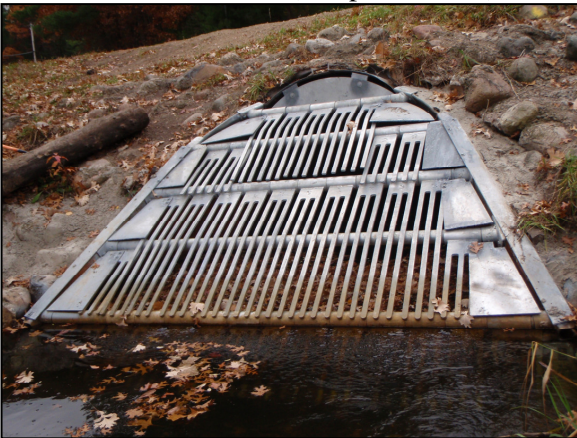
Martin Lake south inlet (completed 2014)
