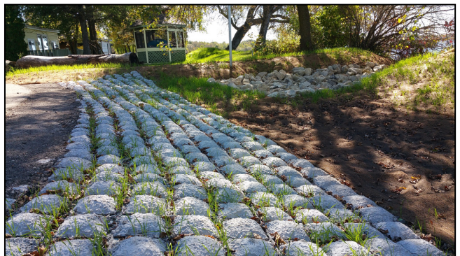
Lincoln Avenue stormwater stabilization.
