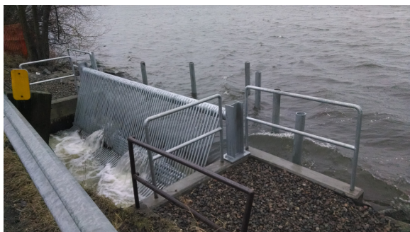
Martin Lake outlet (completed early 2016)
