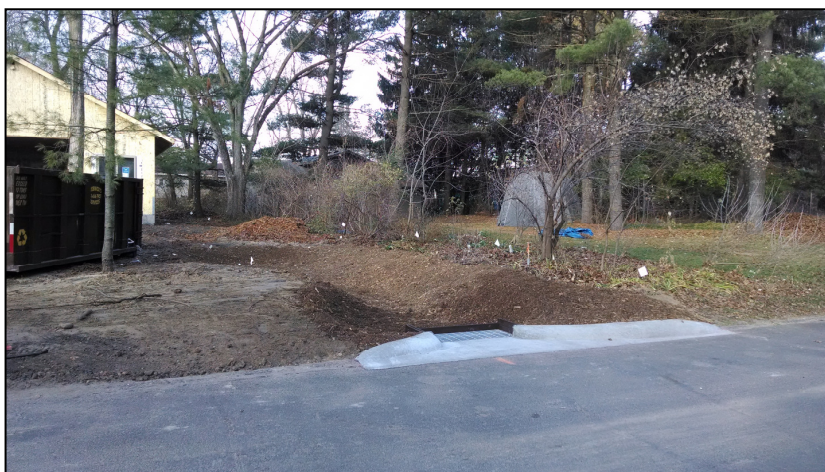
19303 E Front Blvd. NE rain garden to be finished in 2017
