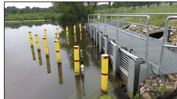
Martin Lake north inlet (completed early 2016)
