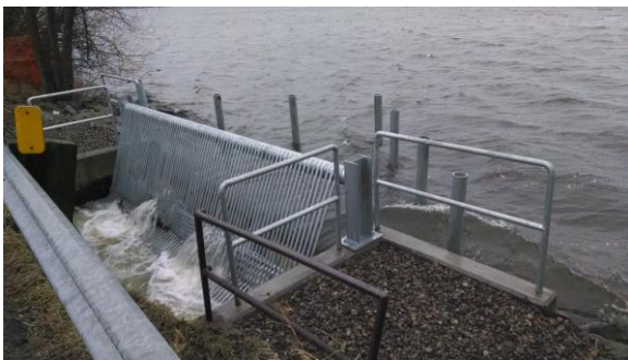
Martin Lake outlet (completion in early 2016)
