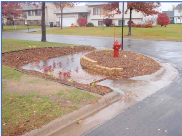
Double-cut rain garden preventing runoff from entering corner catch basin (Area 1).
