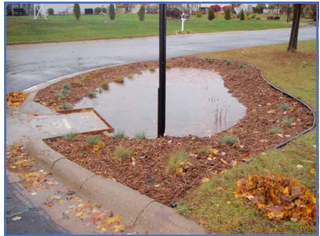
Rain garden near capacity (Area 4).
