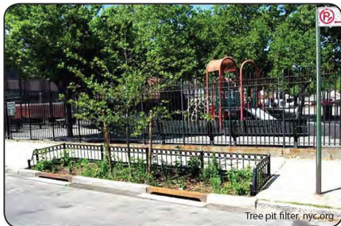
Stormwater tree pits (above) were a recommended treatment option for downtown areas of Cambridge.
