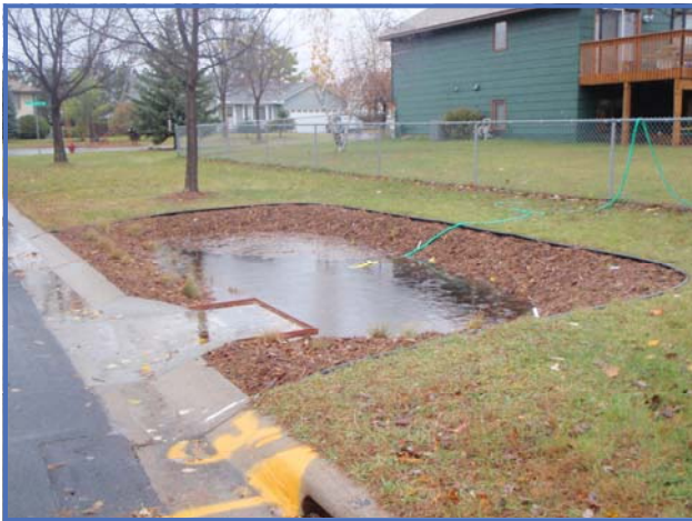
Rain garden upstream of catch basin (Area 3).
